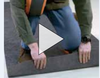
Removal by Hand
