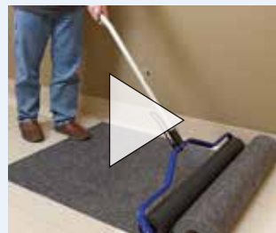
Installation with Roller
